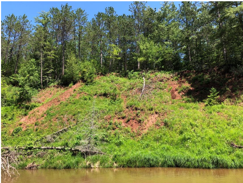
Photo 4. Reach 1, view of steep left descending bank at Transect 7.
