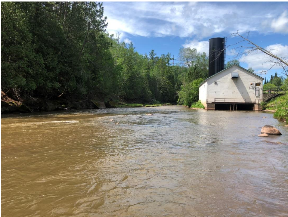
Photo 12. Reach 2, view looking upstream at powerhouse from Transect 10.
