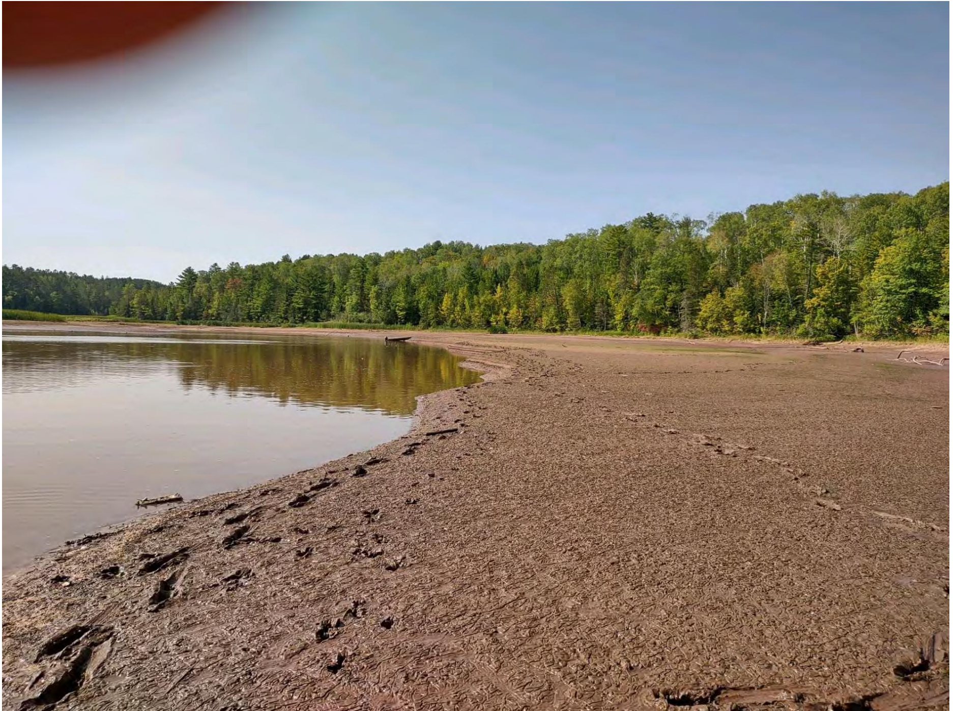
View from dam facing west – September 13, 2022 @ reservoir elevation 705.2'
